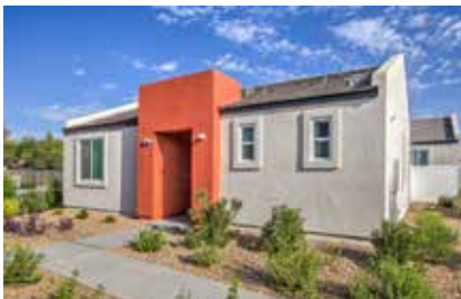
Moderne at Centennial 185 Homes | Las Vegas NV SALE & CONSTRUCTION FINANCING
