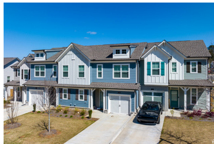
Brighton Townhomes 40 Homes | Acworth GA CONSTRUCTION FINANCING
