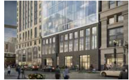
180 W Randolph Hotel mixed-use redevelopment ±0.17 AC CHICAGO, IL
