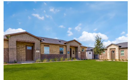
Yardly Dechman 142 Homes | Grand Prairie TX New Construction, Detached Garages IN ESCROW
