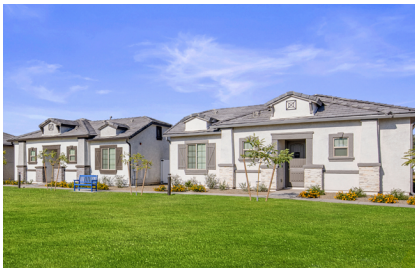
Yardly McDowell 167 Homes | Phoenix AZ New Construction, Detached Garages IN ESCROW
